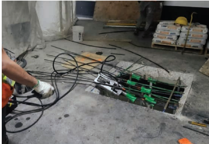
Figure 2: Cables replacement underway in a parking garage
